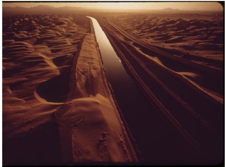
A stretch of the All-American Canal, supplying Southern California with Colorado River water.
