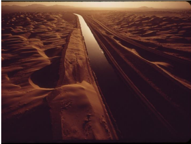
All-American Canal, Colorado River
