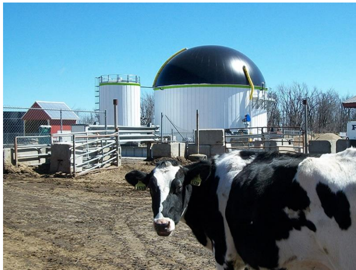
A dairy digester
