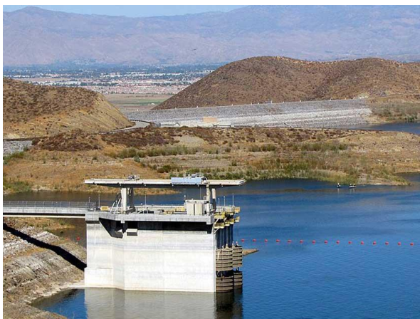
Saddle Dam at Diamond Valley Lake (photo: Lvi56 at Wikipedia Commons)
