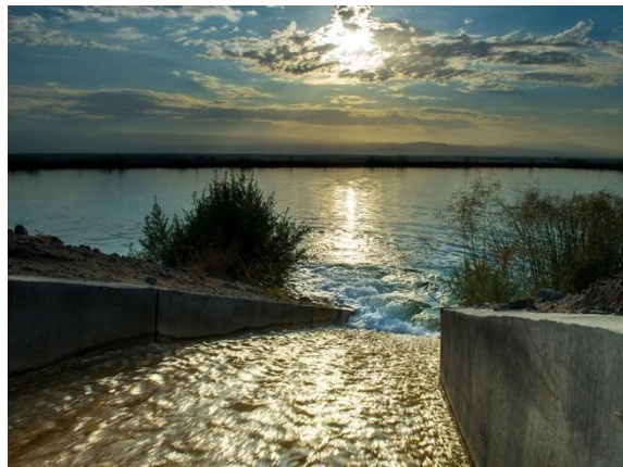
A groundwater recharge pond in the Coachella Valley. (photo: DWR)
