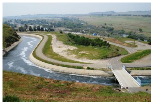
The Friant-Kern Canal sends water to Tulare County farms and communities.
