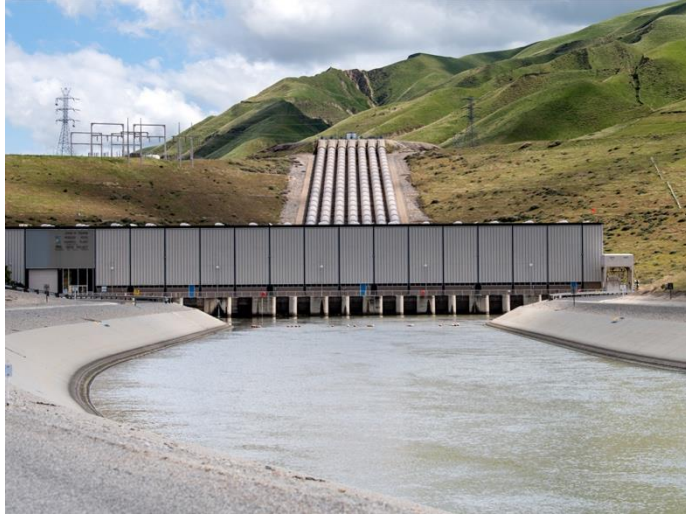
A pumping plant along the California Aqueduct. Courtesy Department of Water Resources
